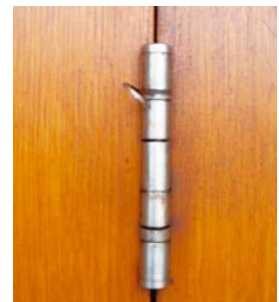
Hinges on high traffic areas which have become badly worn
