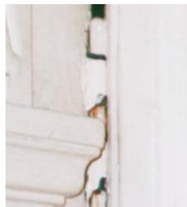
Hinges on high traffic areas which have become badly worn
