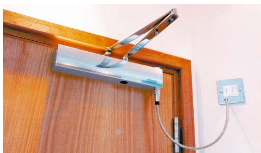
Electro-hydraulic hold open door closer
