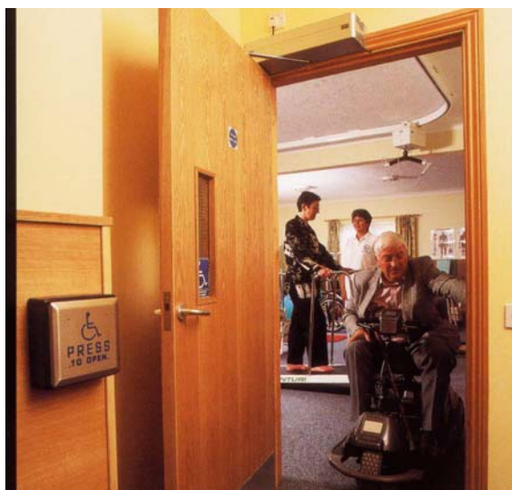
Door automation with a low energy operator
