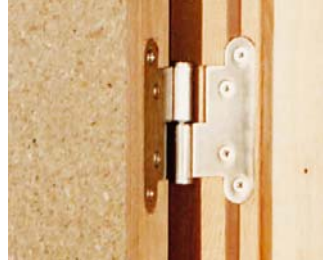
Lift-off hinge
